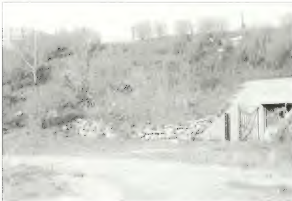
Figure 5.95. View looking northeast at the western side of Battery Mills, circa 1950s. Adding randomly and loosely placed course stones at the toe of the battery's slope would be consistent with a component of its historic appearance. This image shows a stacked stone wall near one of the battery's entries (GATE 20536).
